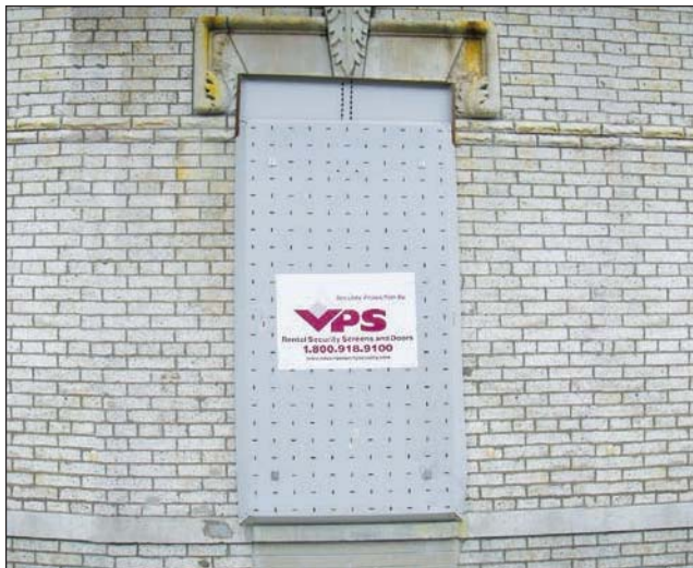
Fig. 12–62. Metal window enclosures
