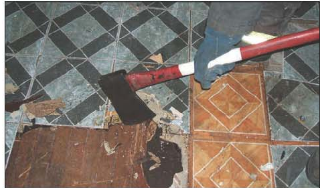
Fig. 12–68. Axe opening a floor
