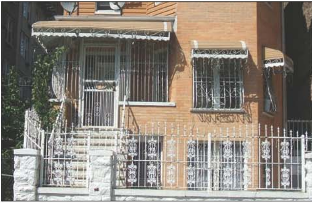
Fig. 12-58. Window bars on a house
