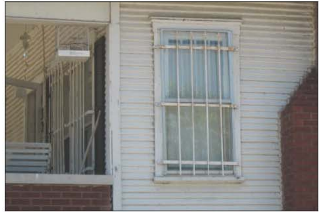
Fig. 12-61. Burglar bars on a wooden frame
