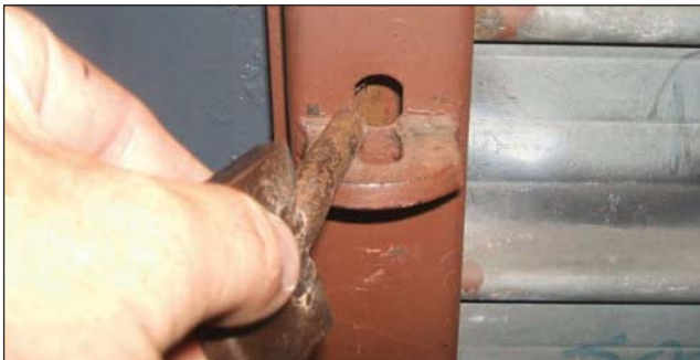
Fig. 12-47. Pin in roll-down gate
