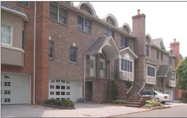
Fig. 14–78. Garden apartments. Garden-type structures, whether residential or commercial, have units that open directly to the exterior.
