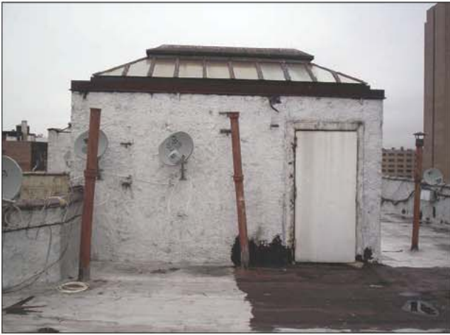
Fig. 14–20. Sometimes we need to be creative when gaining access to vent.
