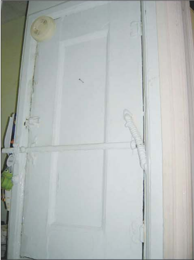
Fig. 14–25. A dumbwaiter shaft door inside an apartment.
