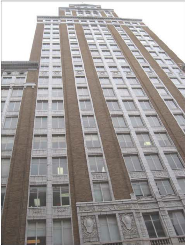
Fig. 14–81. A high-rise office building. Of the various types of structures encountered by the fire service, high-rises can be the most challenging for firefighters to perform ventilation operations.
