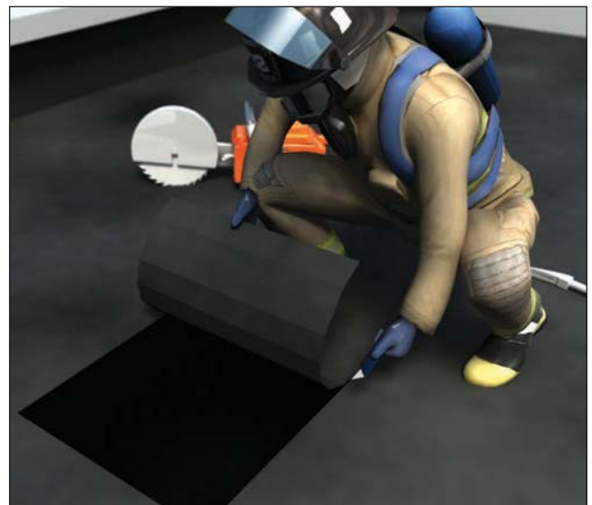
Fig. 14–52. A firefighter using a knife to remove roof membrane to avoid having rubberized material bind the rotary power saw
