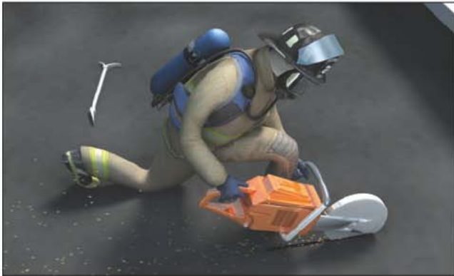
Fig. 14–56. The Kerf cut is a quick way to make an inspection hole during roof operations.
