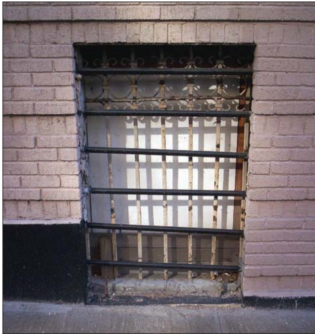
Fig. 14–33. Window bars vary. Some are flush mounted, some are recessed. Look at your district and consider which tools and techniques can negate these security devices.
