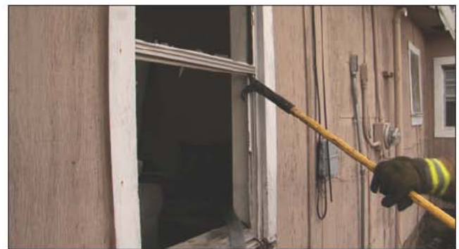
Figure 14–27. Trimming the window by removing remaining glass shards with a tool.
