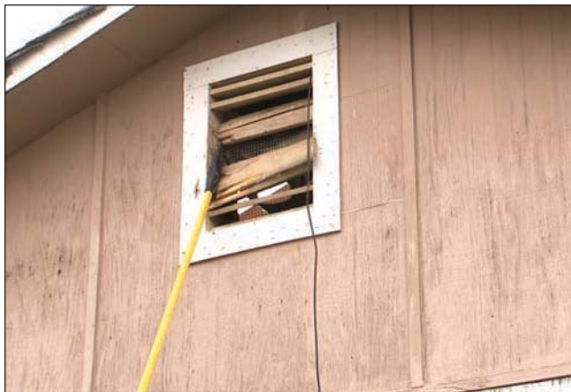
Fig. 14–62. A gable vent being opened for a concealed space helps the ventilation process.
