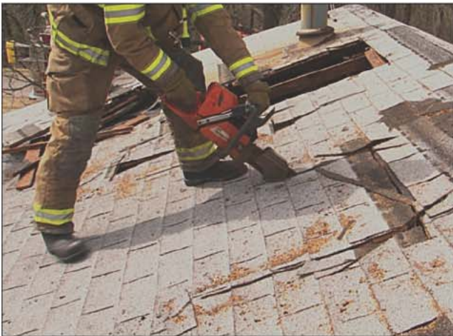
Fig. 14–6. A firefighter venting a roof with a saw.
