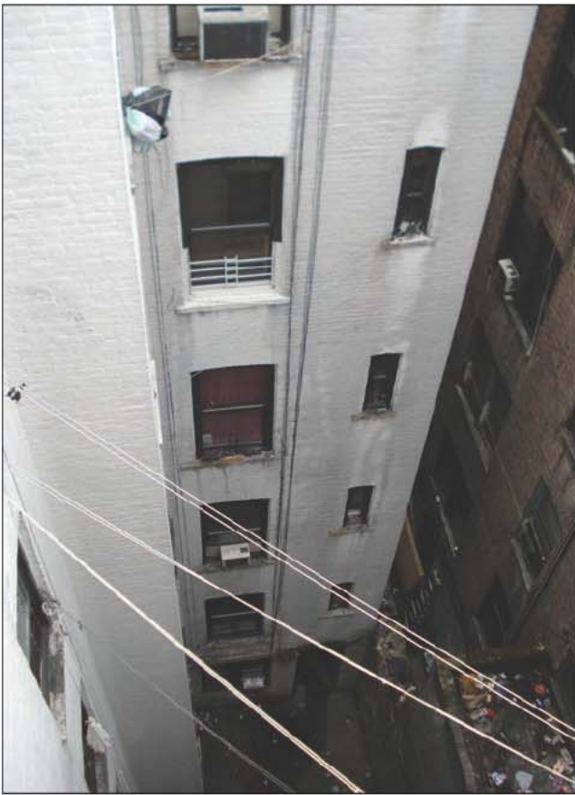
Fig. 14–16. An exterior light well may be used to aid in ventilation provided upper story windows are closed prior to venting.
