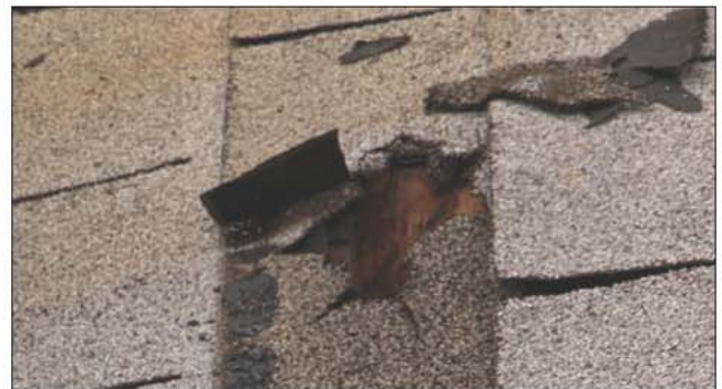
Fig. 14–55. An inspection hole punched in an asphalt shingle roof.
