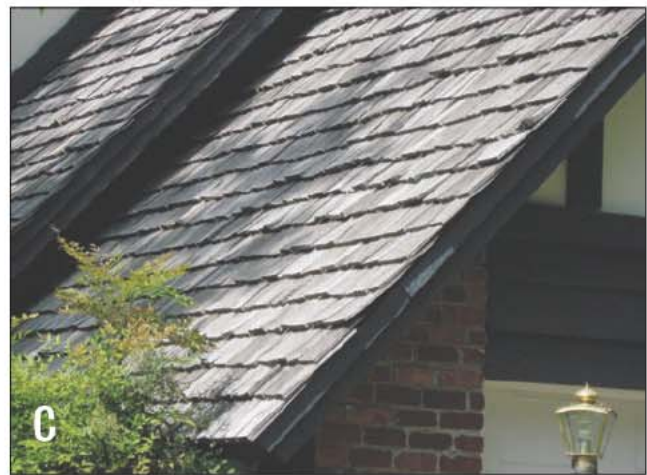
Fig. 14–3. a) Clay tile roof b) Slate roof c) Wood shingle roof
