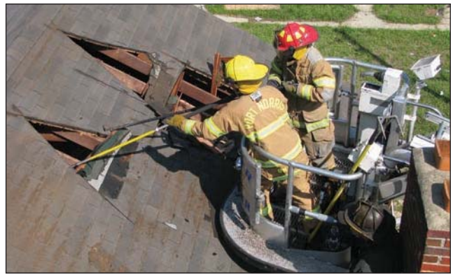
Fig. 14–58. Roof sheathing is removed after a teepee cut has been made.
