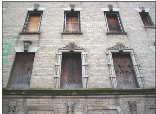
Fig. 14–34. Use a prying action with the Halligan to remove plywood/OSB that has been nailed or screwed into window frames.
