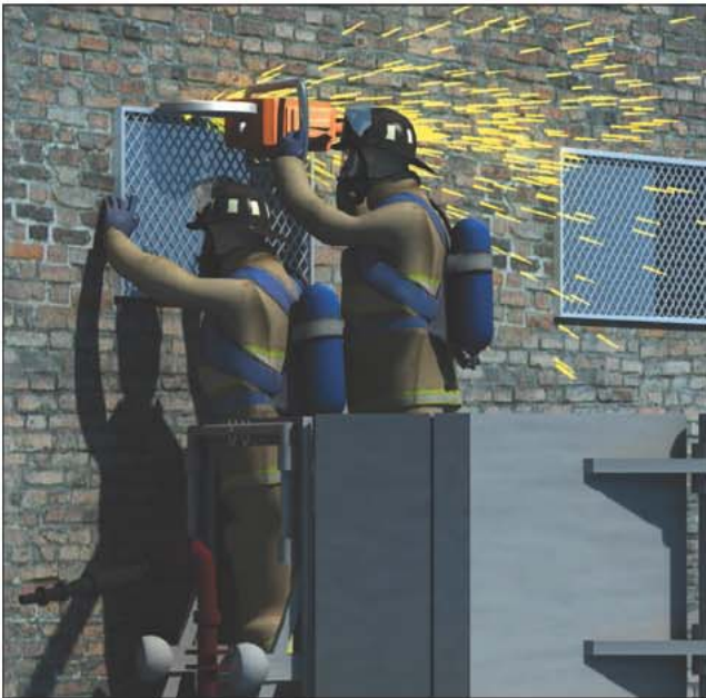
Fig. 14–32. Firefighters use a power saw to cut attachment points of mesh grate to ventilate windows at a one-story commercial building. The tower ladder bucket facilitates the operation.
