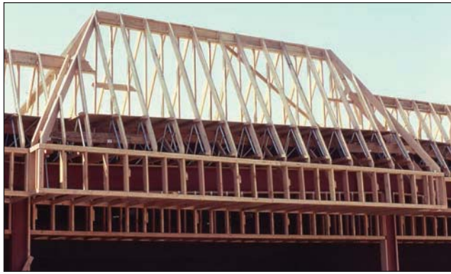
Fig. 14–79. Many commercial occupancies have fascias attached to the front of the building and it may hide the actual age of the building. Consider a fascia to be an additional common attic built onto the exterior wall of the building.
