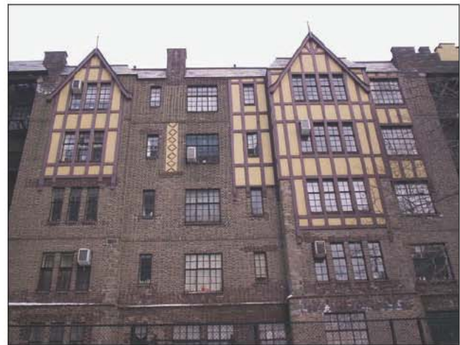
Fig. 14–36. These casement windows on this Tudor-style multiple dwelling will be difficult to force.
