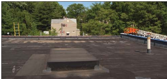
Fig. 14–49. A good practice is to set up an additional ladder as a second means of egress from the roof in case access to the primary ladder is compromised.
