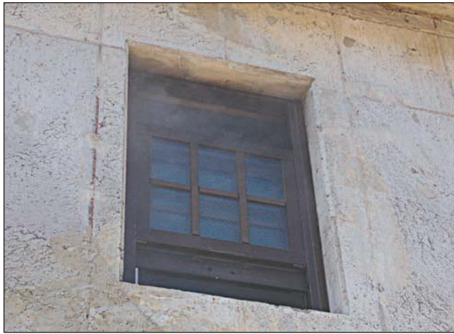
Fig. 14–14. A double-hung window opened two-thirds down from the top and one-third up from the bottom
