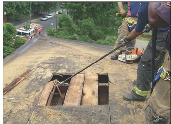
Fig. 14-43. Pulling roof boards with a Halligan hook
