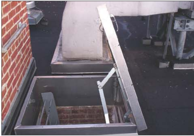
Fig. 14–22. A roof scuttle with a fixed access ladder
