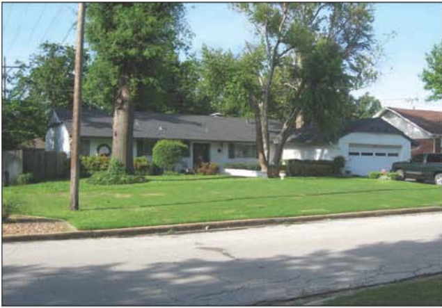
Fig. 14–71. Single story, single-family dwellings are usually accessible; however, indiscriminate horizontal ventilation should be avoided. Always size up and follow your plan.
