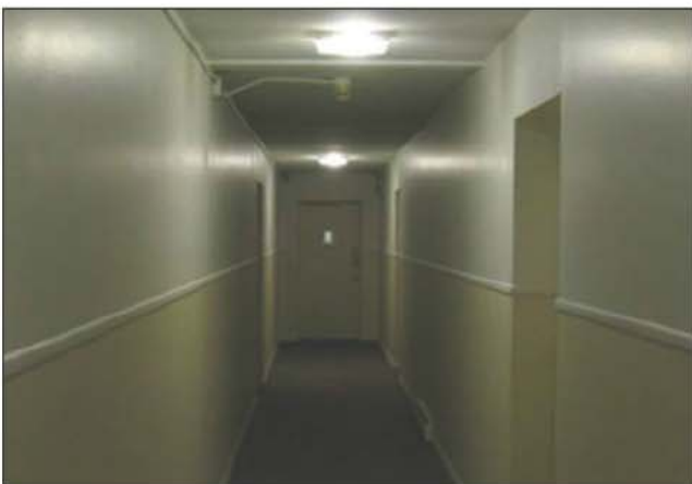
Fig. 14-76. Multiple dwelling and center-hallway buildings. A prior knowledge of these types of buildings in a specific district is essential for firefighters to learn. (Courtesy of Ed Evers)
