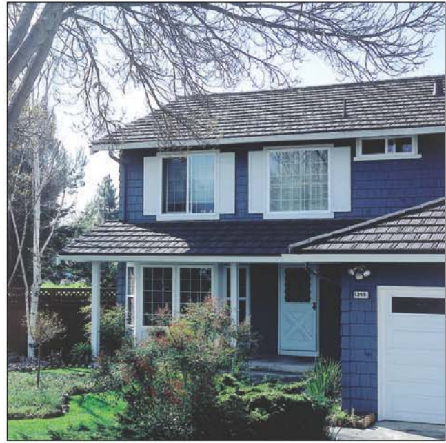
Fig. 14–69. Lightweight steel-tile roofs are often comprised of stone coated interlocking panels of 26-gauge steel that are nailed to 1 x 4 in. (24 x 102 mm) wood battens nailed to an existing or new roof. (Courtesy of Jim Plaster)
