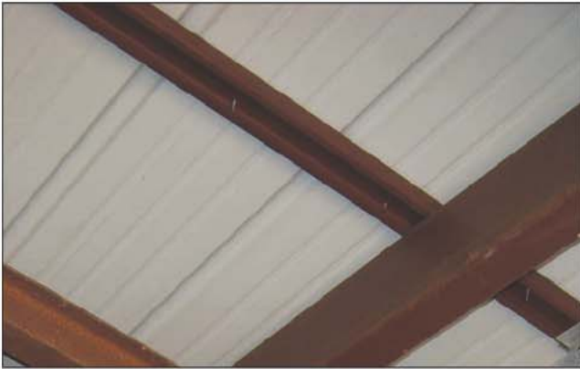
Fig. 14–68. A “C” joist
