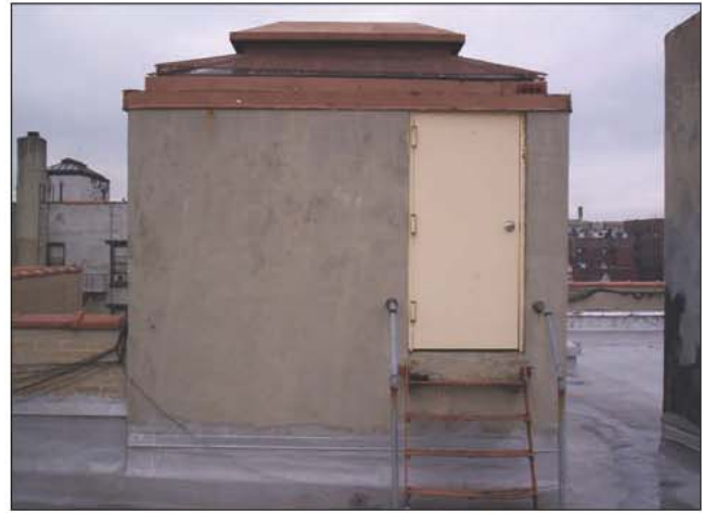
Fig. 14–21. Bulkhead and penthouse
