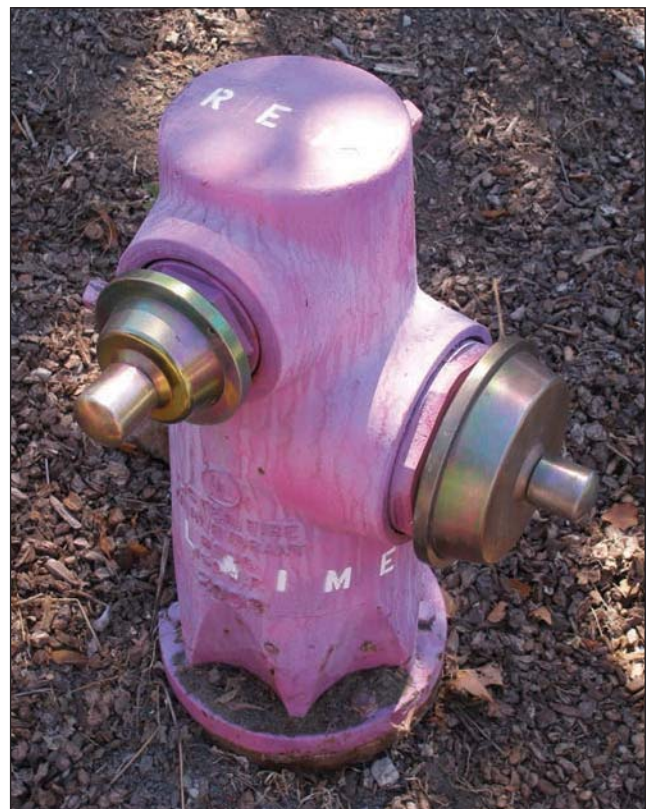
Fig. 15–23. Reclaimed water wet barrel hydrant
