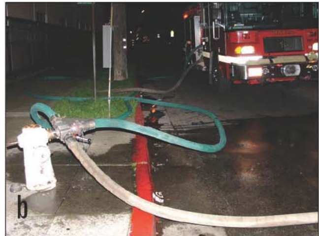
Fig. 15–77. a) Diagram of a typical forward lay. b) Engine pumps through a four-way hydrant valve.
