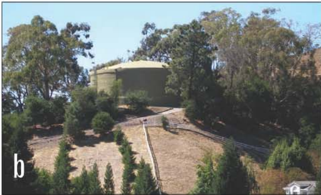
Fig. 15–9 a, b. These treated water tanks use gravity to supply the municipal water supply.
