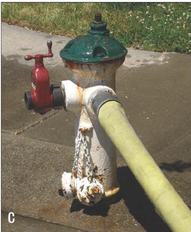
Fig. 15–84 a, b, c, d. From left to right: a four-way hydrant valve, a gate valve, a Carlin automatic hydrant valve, and a Gleason pressure-reducing valve.
