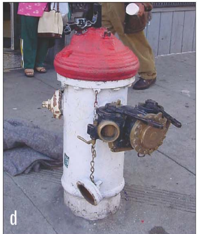
Fig. 15–84 a, b, c, d. From left to right: a four-way hydrant valve, a gate valve, a Carlin automatic hydrant valve, and a Gleason pressure-reducing valve.
