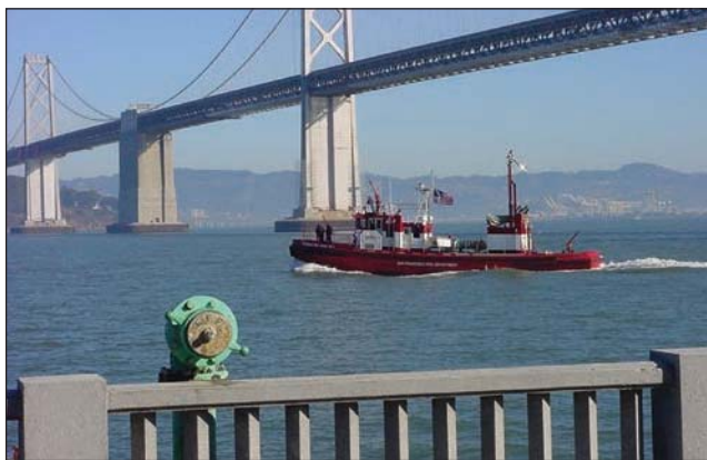
Fig. 15–22. SFFD fireboat Phoenix and waterfront-mounted dry hydrant. (Courtesy of Danny Barlogio)
