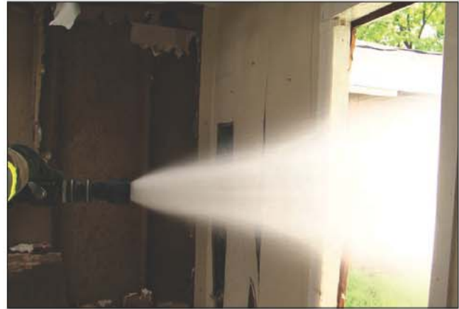
Fig. 16–38. Venting out a window with a fog pattern
