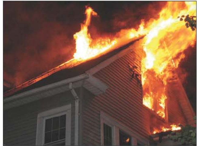
Fig. 17–56. Flashover also indicates signals that the structure itself is under attack from fire.
