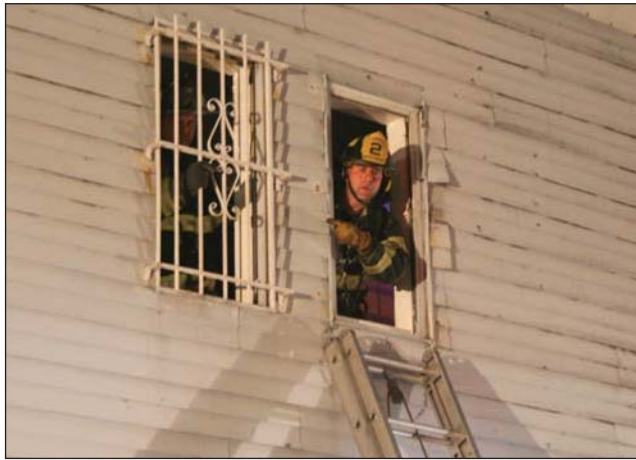
Fig. 17–86. Window bars on wood frame structures are easier to get off from the exterior than from the inside. The firefighter needing to get out may not have the time to remove them from inside the building. Remove them as soon as you see them to avoid critical situations later. (Courtesy of Ron Jeffers)
