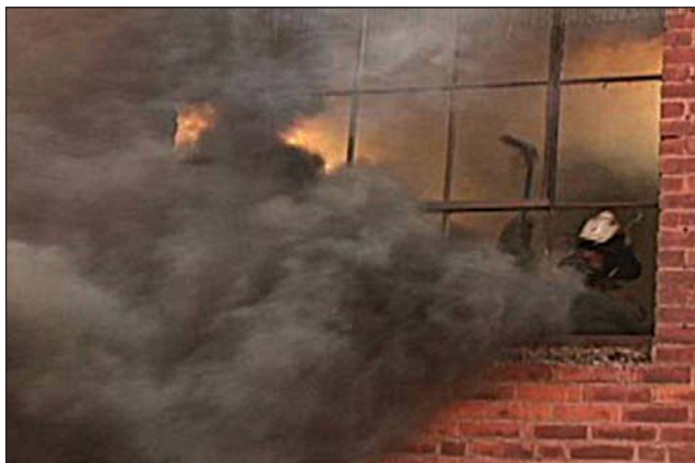
Fig. 17–87. Metal casement windows pose the same hazards as window bars. (Courtesy of Jim Duffy)
