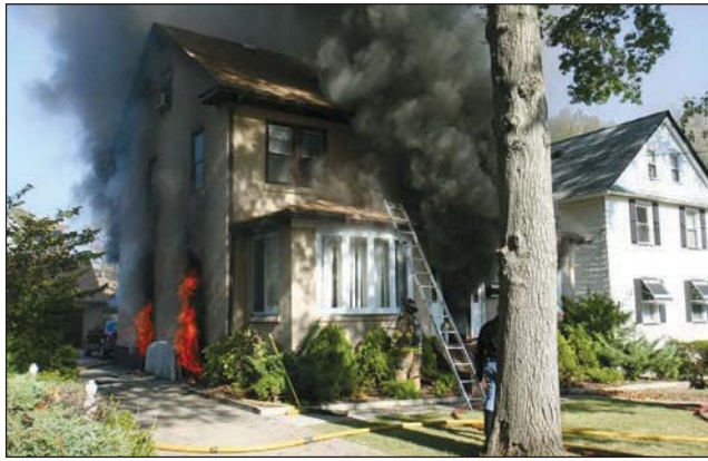
Fig. 17–61. Basement fires have limited ventilation points and offer the greatest chance for extension through voids. (Courtesy of Chris Saraceno)
