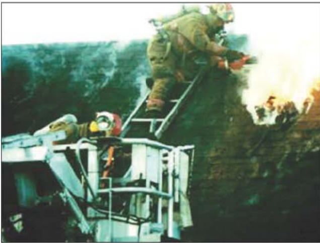
Fig. 17–70. Firefighter wearing full PPE while cutting a hole in roof. (Courtesy of the Middletown, CT, Fire Department)
