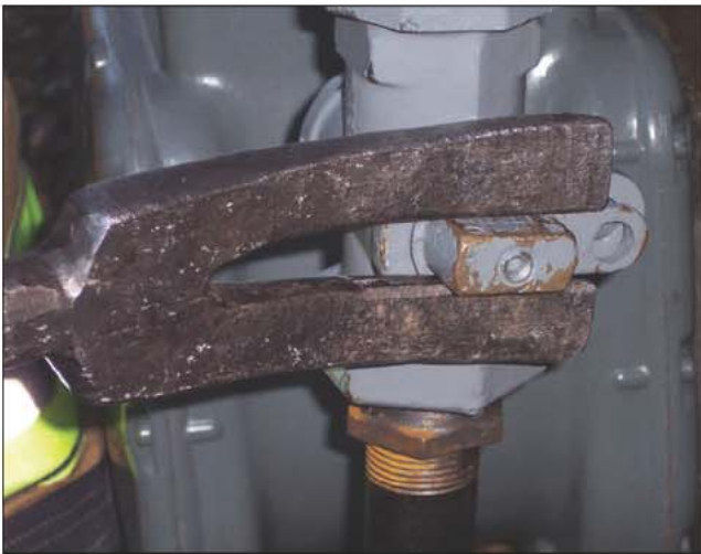
Fig. 17–40. A tool closing a gas cock (perpendicular to flow)
