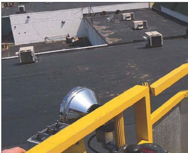
Fig. 17–67. Store depths will vary, making it easy to walk off the roof. Try to cross in the front where they are usually even with the street and sidewalk.
