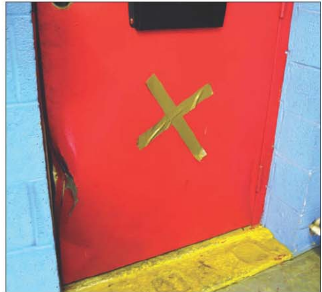
Fig. 19-5. In order to prevent a duplication of effort, it is necessary for firefighters performing a search to mark the room as "searched" in a conspicuous manner, according to local policy.
