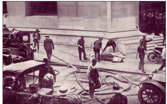
Fig. 2-17. Many Americans think that the terrorist attacks of September 11, 2001, were the first on American soil. There have been many attacks through the country's history, including this one on Wall Street in 1920. Damage to this building's (the J.P. Morgan bank) exterior wall, near the corner of Wall and Broad Streets, is still visible.
