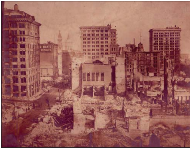
Fig. 2–11. The Great Baltimore Fire of 1904 led to creation of the first comprehensive standardized building code. Firefighters were not successful in standardizing hose threads; many responding mutual aid fire departments, including New York City, were unable to attach their hoses to Baltimore's hydrants. There are still a multiplicity of hose threads across the United States today.
