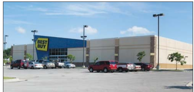
Fig. 20–73. Here a big-box-type construction building houses a retail outlet.
