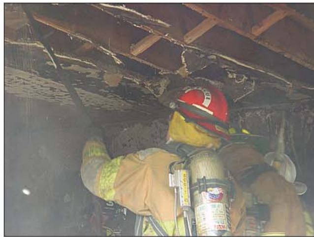
Fig. 20–58. Opening walls and ceilings after the initial fire attack must be done quickly to search for hidden fire. Fire can travel undetected in void spaces and is a serious threat to firefighters. (Courtesy of Tom Bierds)
