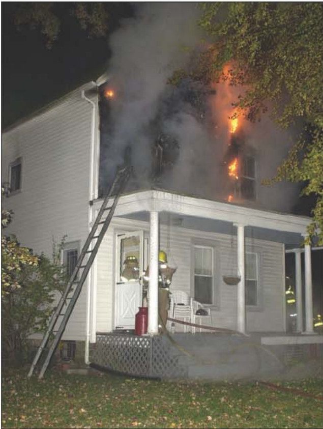
Fig. 20–7. Size-up of this fire reveals that the fire appears to be contained to one or two rooms on the second floor. An offensive attack could result in saving the building and contents with a reasonable risk to firefighters. However, if this building was built with lightweight construction materials, it could be a deathtrap for firefighters. Incident commanders must realize these dangers to firefighters. (Courtesy of Brian Duddy)
