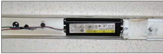
Fig. 20–80. Starter and ballast
