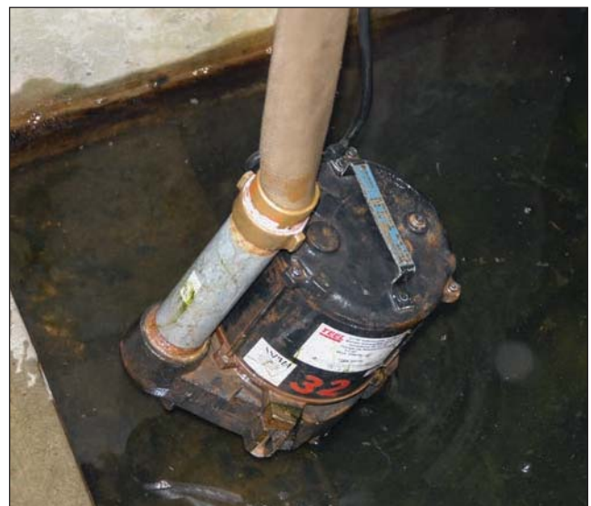
Fig. 21–11. Dewatering pumps should be placed at the lowest collection point so that the water will drain toward the pump.
