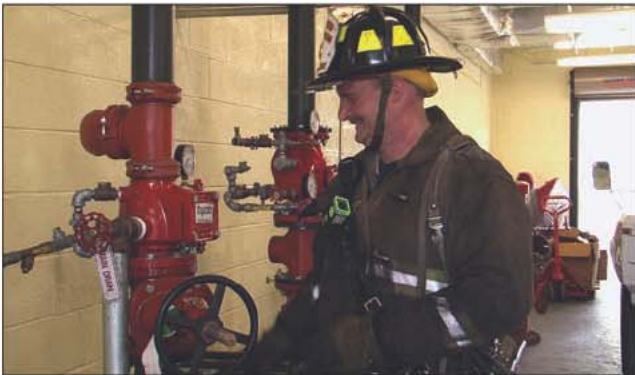
Fig. 21–12. An outside stem and yoke (OS&Y valve) in the “open” position
