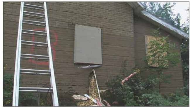
Fig. 21-16. Plywood can be used to secure broken windows.
