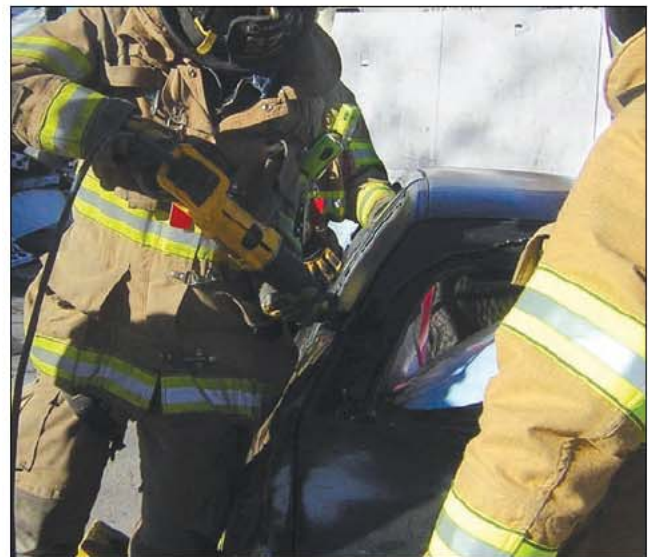
Fig. 34–52. A reciprocating saw used to cut a C Post
