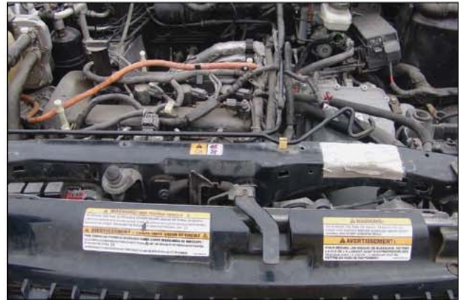
Fig. 34–42. This photo reveals the orange HV cable in the engine compartment of the 2007 Escape Hybrid.
