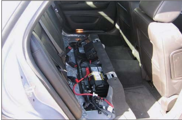
Fig. 34–11. As previously mentioned, batteries may be located in many locations such as under the rear seat found in the 2007 Cadillac CTS .
