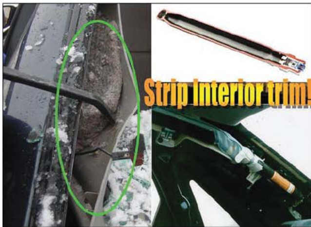
Fig. 34–53. Always strip trim to find side curtain cylinder before cutting a roof or post.
