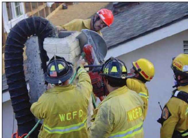
Figs. 35–74 and 35–75. Even a person trapped inside a chimney constitutes a confined space rescue and may require specialized equipment.
