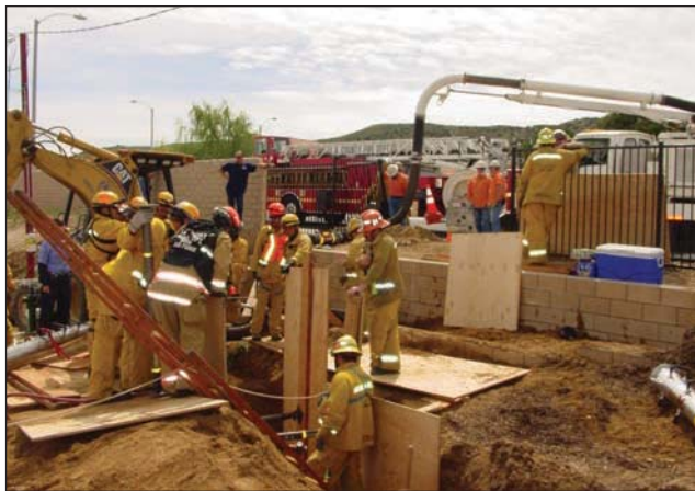
Fig. 35–57. Emergency vehicles should be staged at least 50 ft away from trenches.
