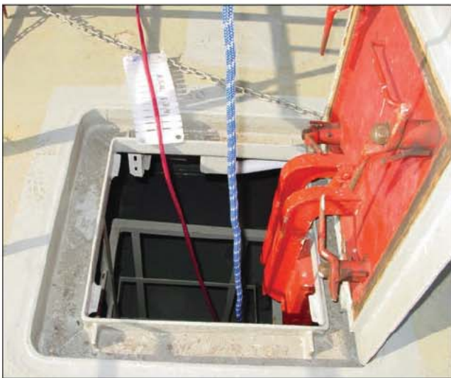
Fig. 35–63. Underground vaults are merely one example of confined spaces.
