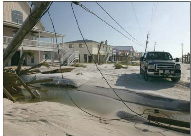
Fig. 35–103. Downed power lines
