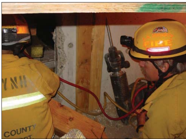
Fig. 35–37. Assisting technical rescue teams by supporting breaching, breaking, and forcible entry operations is a common task for the firefighter.
