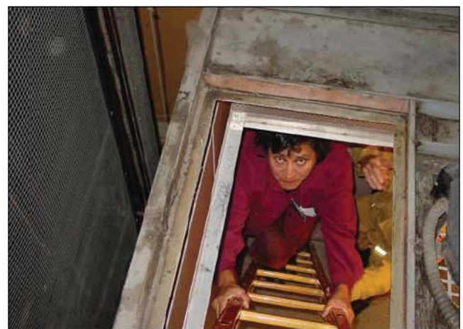
Fig. 35–88. Victims using a ladder to evacuate an elevator car should be assisted by firefighters and given direction.
