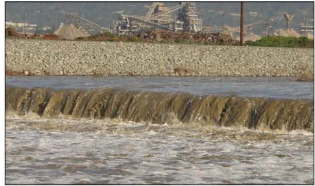
Fig. 35–7. Low-head dams should be treated with great caution as they can be potentially dangerous to responders.
