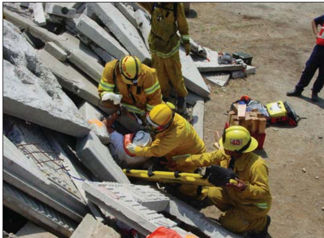
Fig. 35–26. Surface rescue is attempted on the outside of a structural collapse incident and involves rescue victims trapped beneath nonstructural elements.
