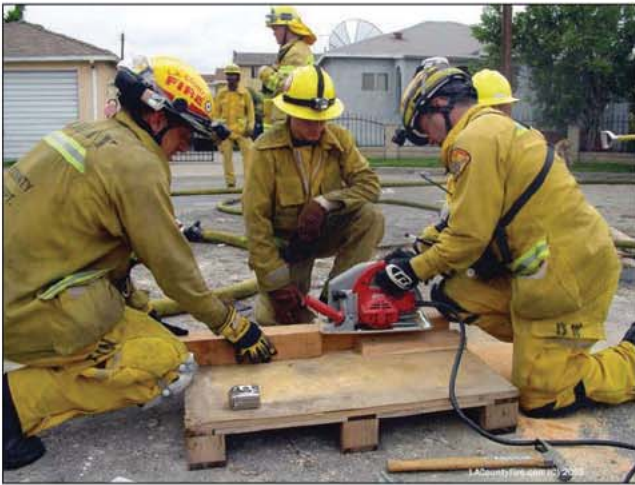
Fig. 35-59. Cutting and assembling lumber at a trench rescue incident will require several firefighters.
