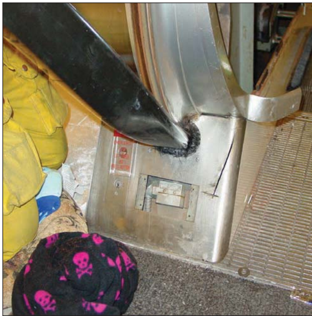
Fig. 35–91. If not already done so by bystanders upon your arrival, the emergency stop switch should be activated.
