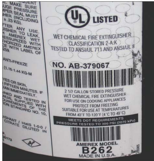
Fig. 6–1. This label from Underwriters Laboratories (UL) certifies that this fire extinguisher has been tested to their rigid standards.
