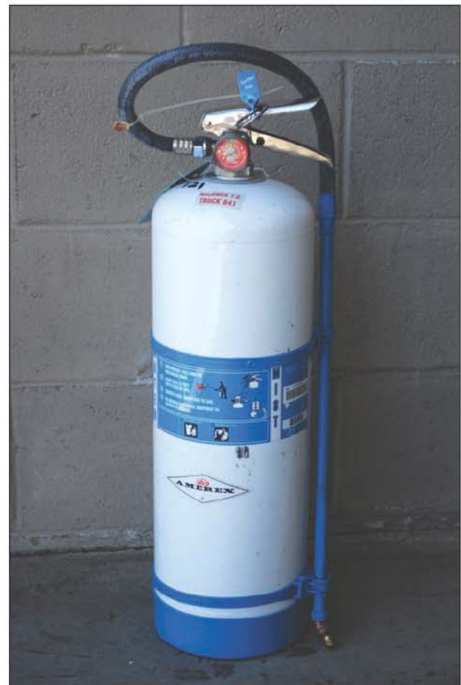
Fig. 6–9. Water mist extinguisher
