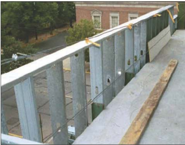
Fig. 7–21. A curtain wall system being installed on a building. The wall panel passes in front of the floor slab and does not support any part of the building other than itself. Curtain walls may be responsible for fire extension between floors if the wall space is not properly fire-stopped at each floor level.
