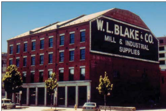
Fig. 7–30. Mill buildings may have large open floor areas and firewalls that sub-divide the floor areas of the building. In the photo, you can see the firewalls extending above the roof of the building. Mill buildings typically had many large openable windows to allow for natural light and ventilation. (Courtesy of Courtney A. Dansbach)
