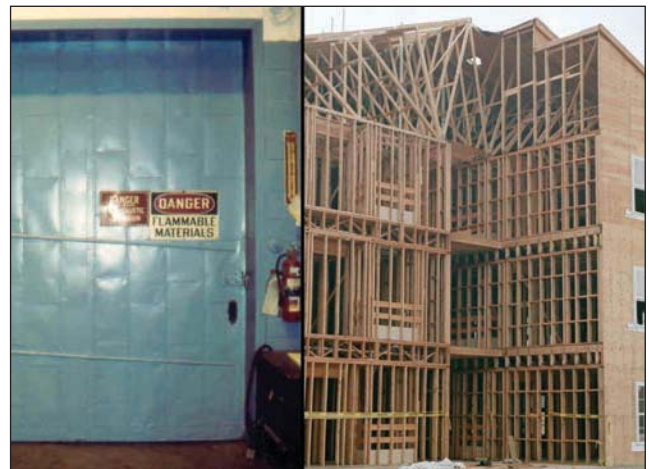
Fig. 7–11. Fire loads will vary from building to building. Flammable liquids, which are used or stored in the building, will present a higher fire load. The wooden structural members of the building also contribute to the fire load.
