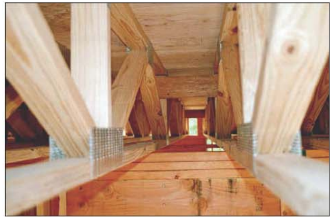
Fig. 7-14. Use of lightweight wood parallel-chord truss members in a floor system. The use of floor trusses creates a large combustible void space. Buildings framed with dimensional lumber, which use 2 in. × 10 in. (51 mm × 254 mm) floor joists, will not have this combustible void space.
