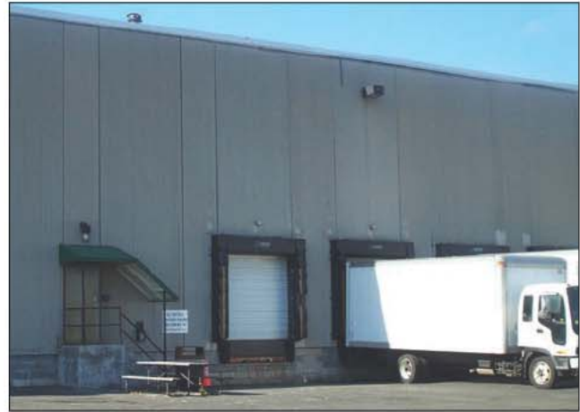
Fig. 7–25. Exterior tilt-slab wall of a noncombustible warehouse occupancy. In tilt slab construction, the exterior wall system relies on the roof for support. If a fire causes the roof to collapse, there is a tremendous likelihood that the walls will collapse next.
