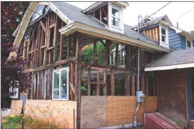
Fig. 7-32. This photo details a post and beam building. Notice the vertical post at the corners and the horizontal beams at the floor level. (Courtesy of Tim Hetzel)
