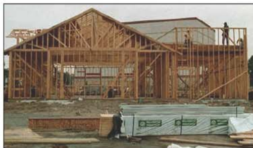
Fig. 7-1. A wood frame building
