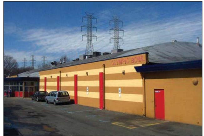
Fig. 7–27. Common ordinary-constructed buildings that are constructed with truss roofs include bowling alleys, automobile dealerships, gymnasiums and churches. In this photo, you can identify the strong areas of support in the brick columns built into the exterior walls. (Courtesy of Christian P. Dansbach)
