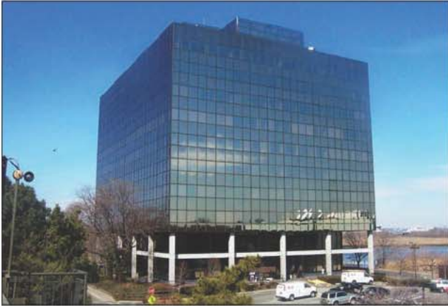
Fig. 7–24. This office building is a non-combustible constructed building with a glass curtain wall system. This wall system makes identifying the number of floors in the building extremely difficult if not impossible from the exterior.
