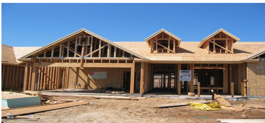
Figure 3. Lightweight Construction Truss System
