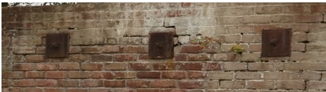
Figure 31. Post 1959 Masonry Construction Rafter Tie Plate
