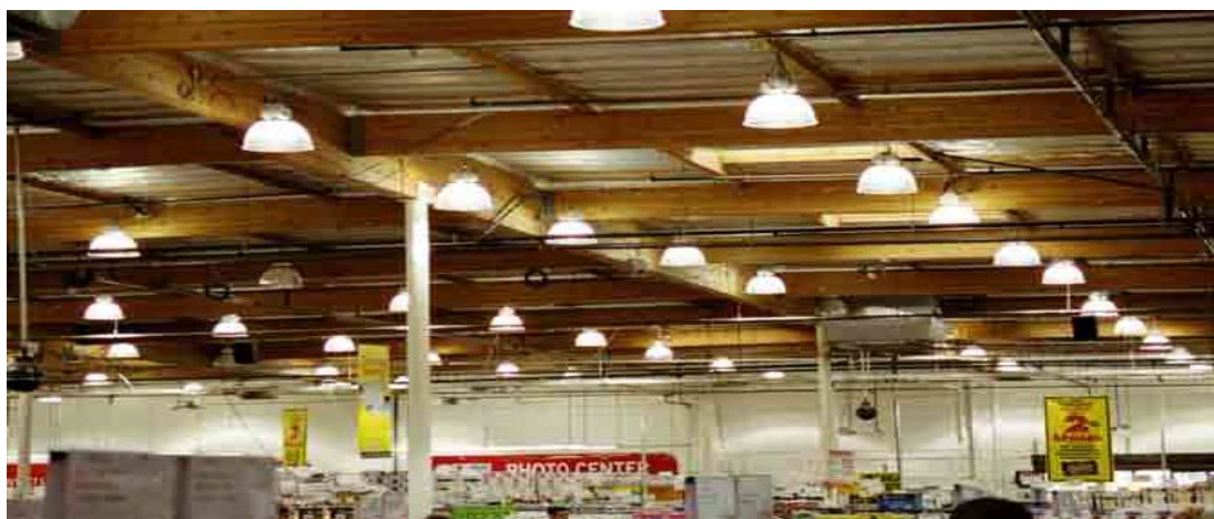
Figure 20. Panelized Roof
