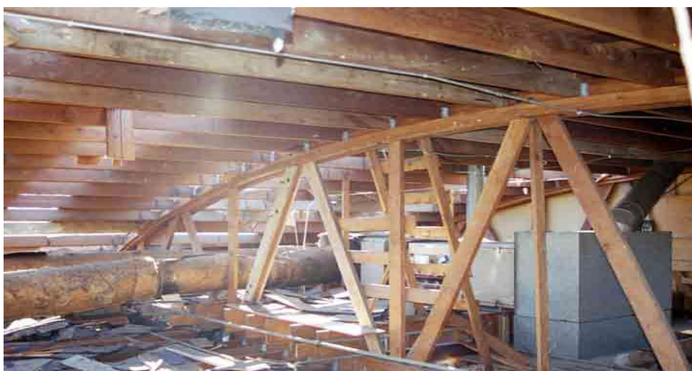
Figure 11. Bow String Construction
