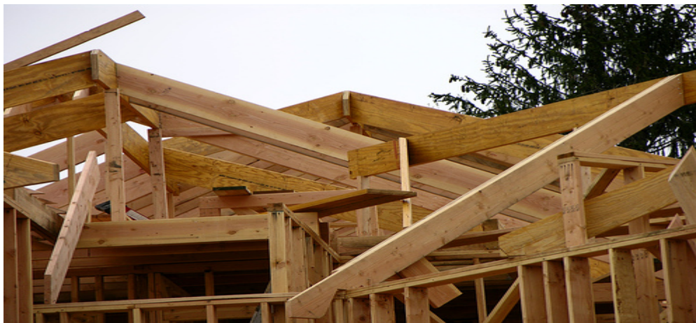
Figure 7. Conventional Construction Gable Roof
