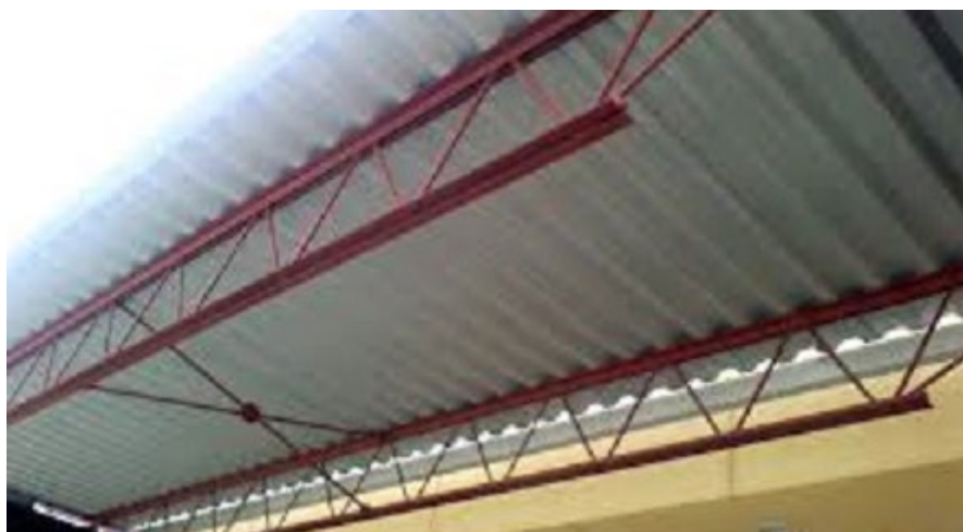
Figure 17. Open Web Truss
