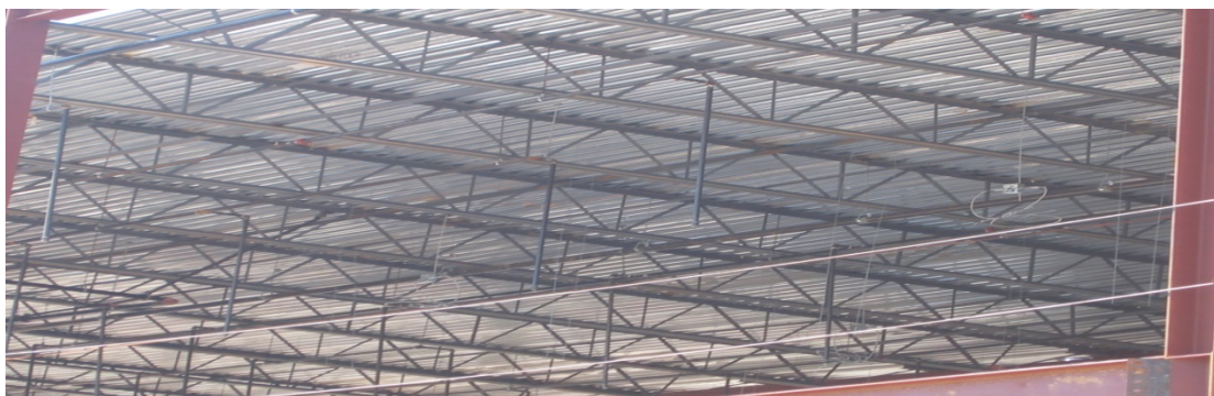
Figure 26. Corrugated Metal Roof
