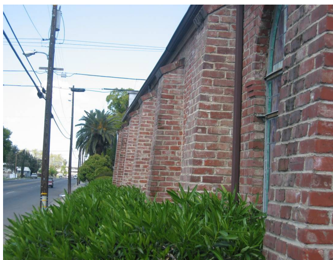
Figure 29. Unreinforced masonry building
