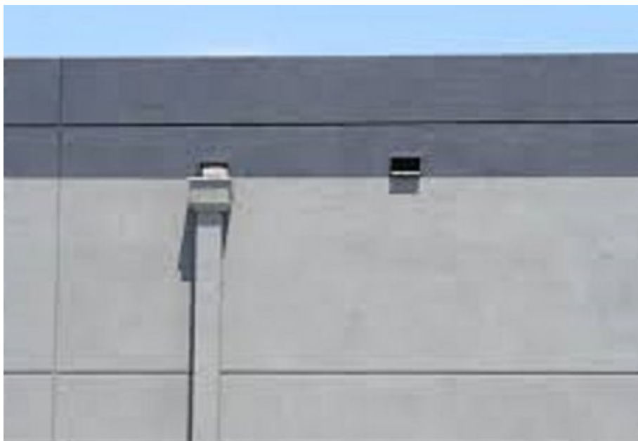
Figure 39. Scuppers with Parapet Wall
