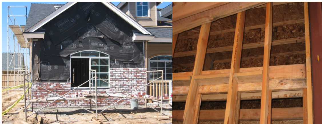
Figure 35. Frame Construction and Fire Blocks
