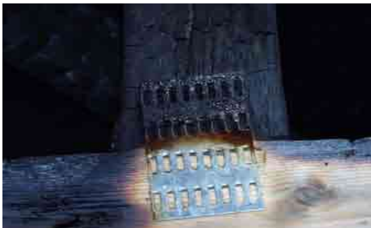
Figure 18. Metal Gusset Plate
