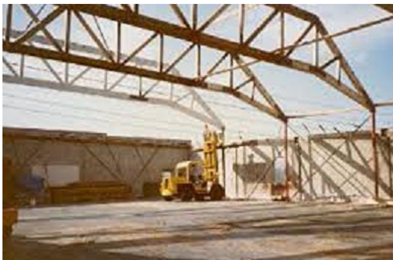
Figure 10. Sloping Ends of Bridge Truss
