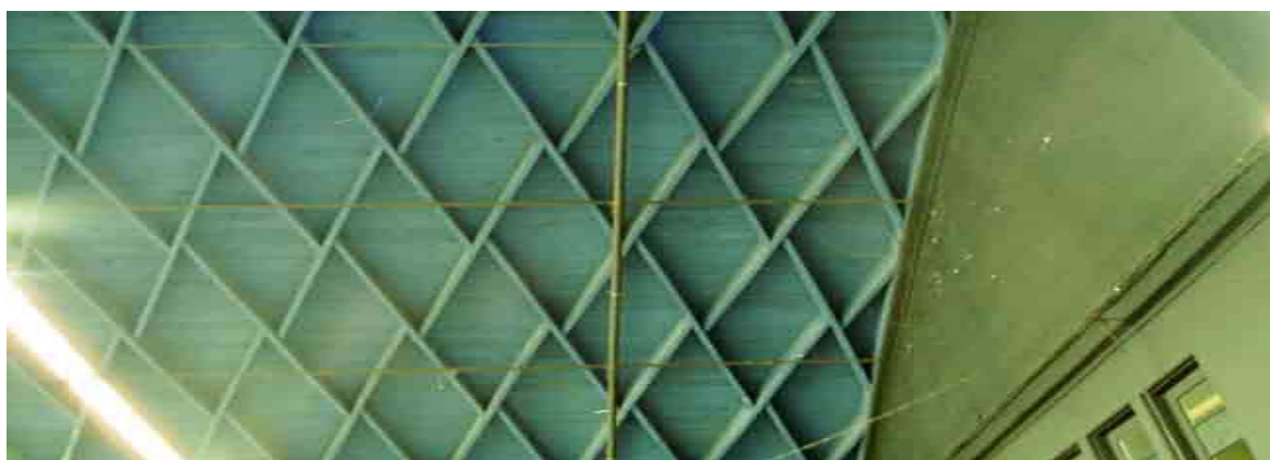
Figure 12. Lamella Arch Roof
