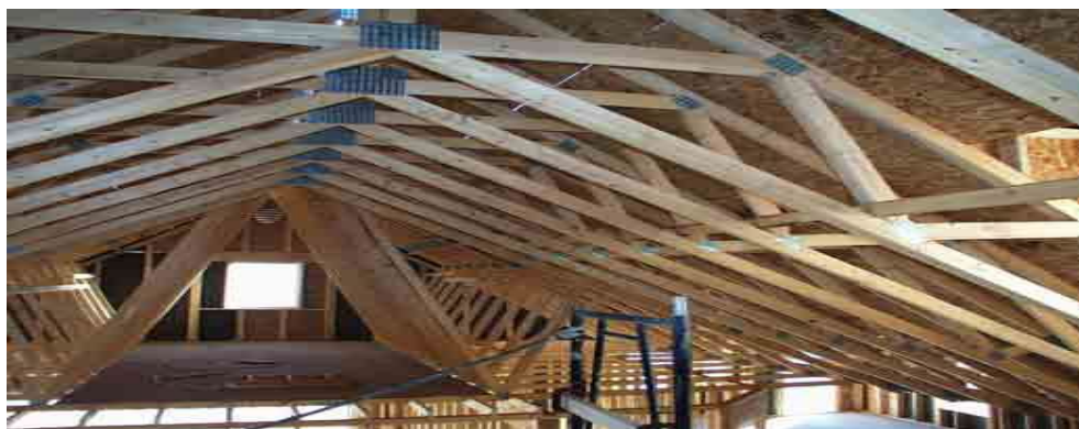
Figure 19. Metal Gusset Truss System
