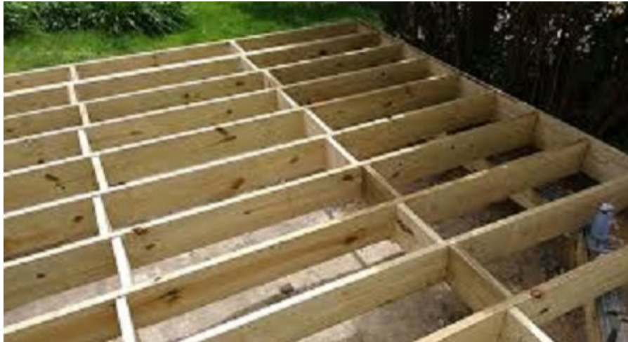
Figure 16. Nailing Blocks
