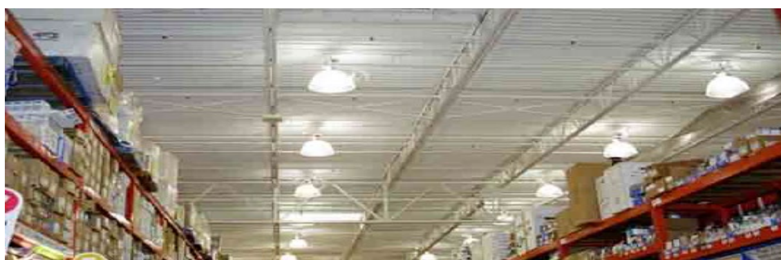
Figure 24. Open Web/Parallel Truss
