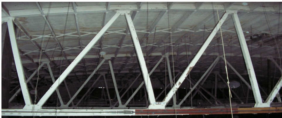
Figure 9. Bridge Truss Roof
