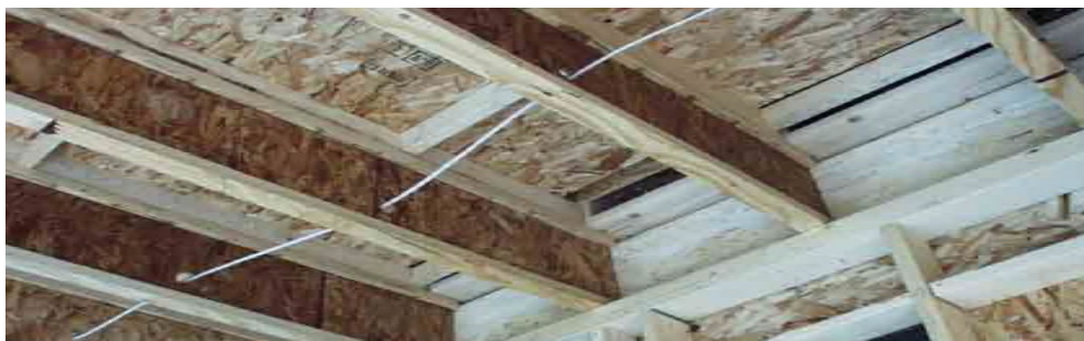
Figure 15. Wooden I Beam Roof
