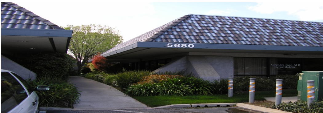
Figure 36. Large Facade with Overhang
