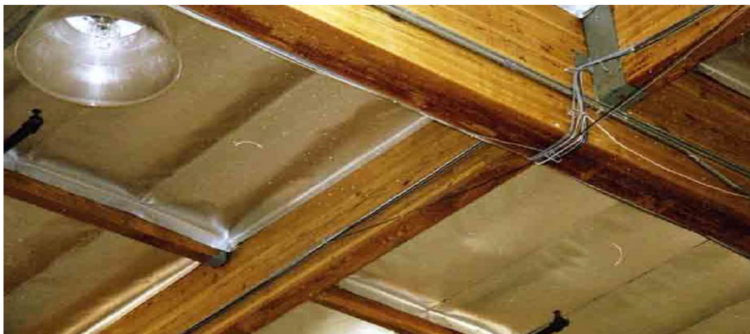
Figure 22. Panelized Roof, notice the nailing blocks and joist hangers
