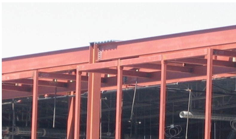
Figure 27. Metal Beam Structural Members
