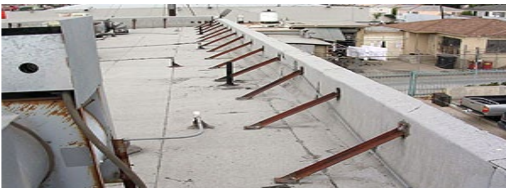
Figure 34. Steel Bracing Added to Parapet Walls
