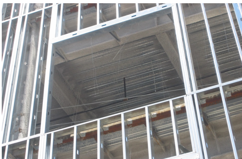
Figure 43. Curtain Construction Glass Opening
