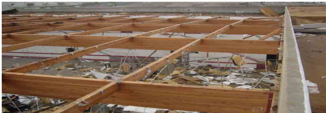
Figure 21. Panelized Roof Framing
