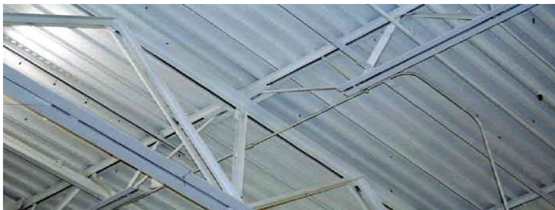
Figure 23. Open Web/Parallel Truss
