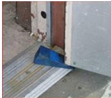
Figure 108 - Place wedge out of the walking path so it does not get kicked out
