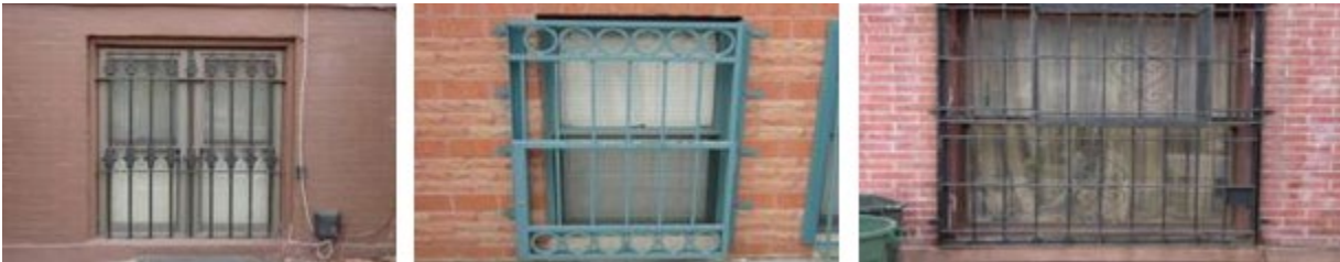
Figure 198 - Security bars in masonry
