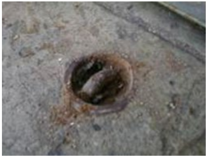
Figure 183 - Examples of locking devices found on roll-down gates
