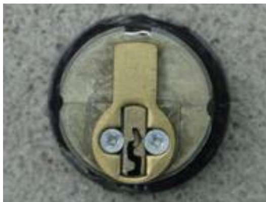
Figure 140 - Lock cylinder removed
