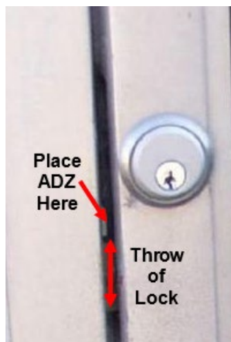
Figure 151 - Throw of lock is down
