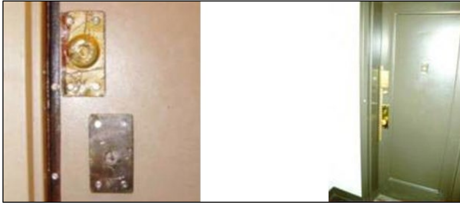
Figure 46 - Angle iron over door gap
