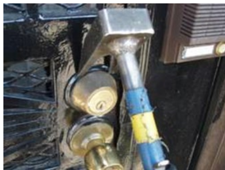
Figure 123 - Remove cylinder
