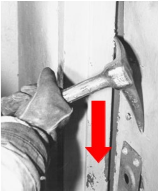
Figure 52 - Gap the door up and down
