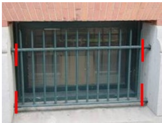
Figure 201 - Utilize the rotary saw to cut the bars off
