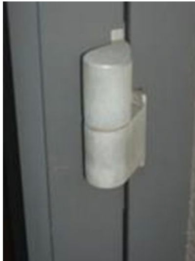
Figure 98 - Pin type hinge
