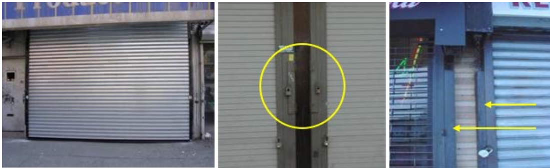
Figure 181 - Notice the different housing for the pull chain
