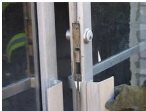
Figure 149 - Completed cut on pivoting bolt
