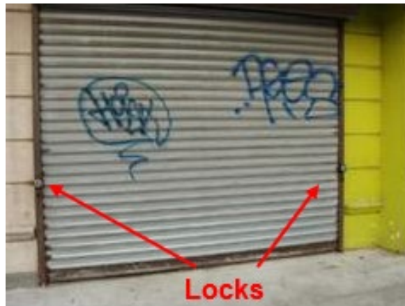
Figure 178 - Exterior locks on roll up door/curtain
