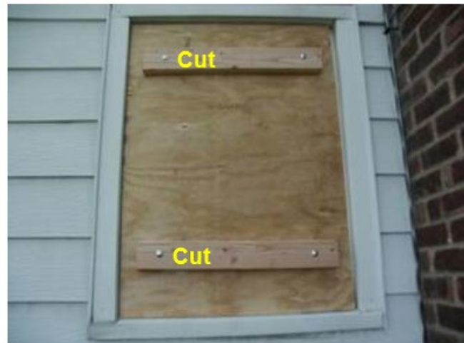
Figure 212 - Cut the bolt heads with a rotary saw
