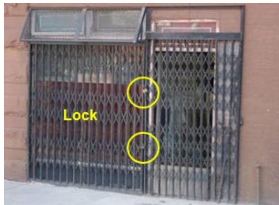
Figure 173 - Sliding scissor security gate
