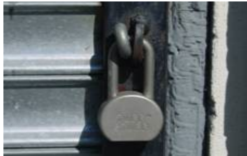
Figure 185 - Padlock through a pin bolt
