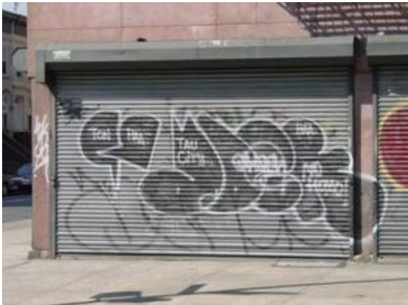
Figure 180 - Mechanical roll down gate (Chain Hoist)
