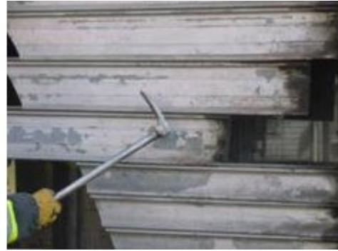
Figure 194 - Drive pike into slat to remove sections
