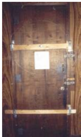
Figure 43 - Double drop bar
