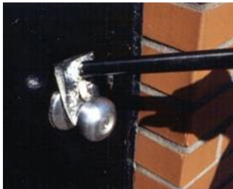
Figure 116 - Knob removal
