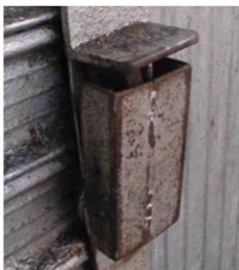
Figure 190 - Examples of external shields around locks
