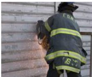
Figure 196 Cutting the roll down curtain
