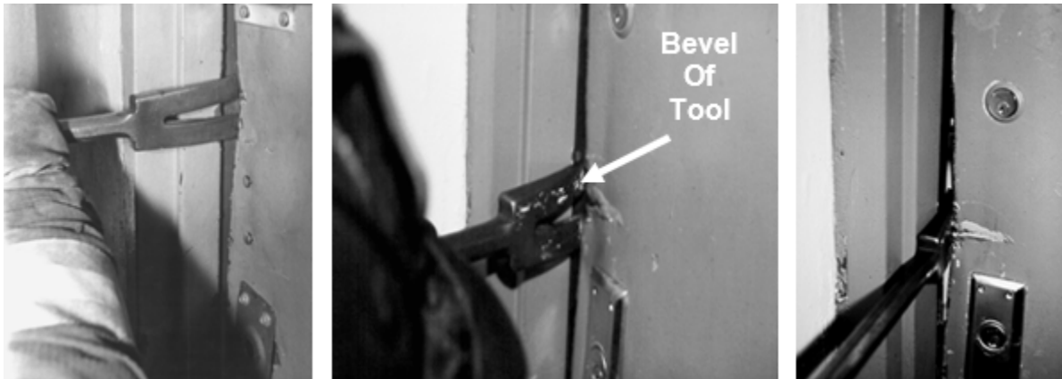
Figure 53 - Gap the door
