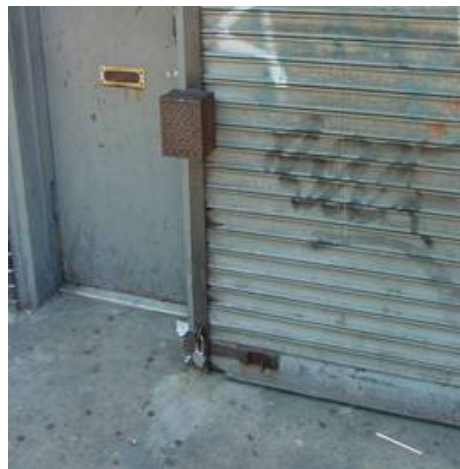
Figure 160 - Tank lock
