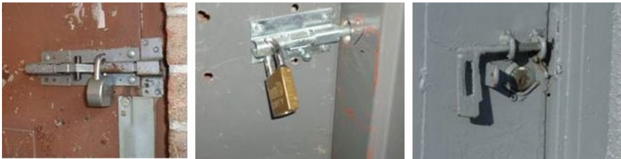
Figure 42 - Slide bolt added on with supplemental locks
