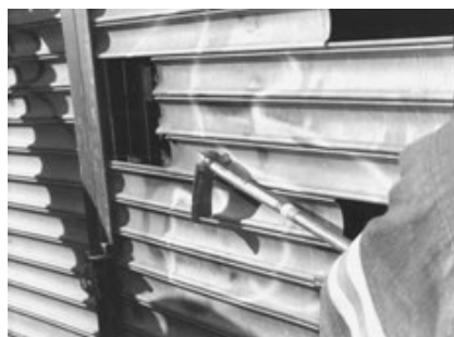
Figure 197 - Drive the Pike end of the Halligan into a slat to remove. If slats are tight, drive the Halligan with an axe.
