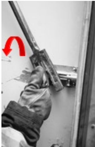
Figure 163 - Twist slide bolt off with the fork of the halligan
