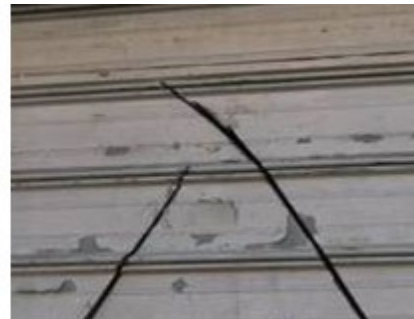
Figure 193 - Do not cross cuts until second cut is complete
