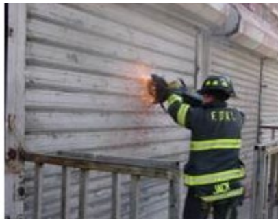
Figure 193 - Do not cross cuts until second cut is complete
