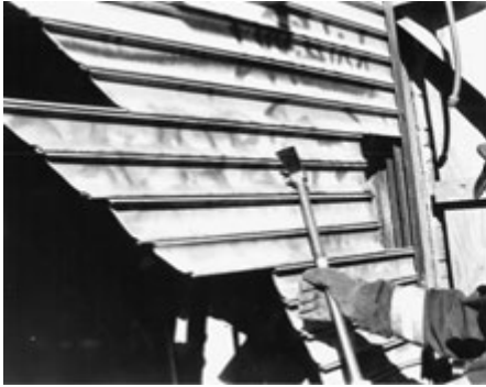
Figure 194 - Drive pike into slat to remove sections
