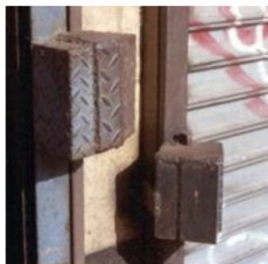
Figure 190 - Examples of external shields around locks
