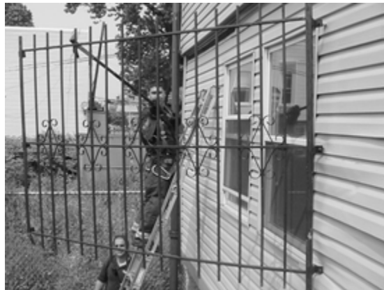
Figure 202 - Swing the bars away from the window
