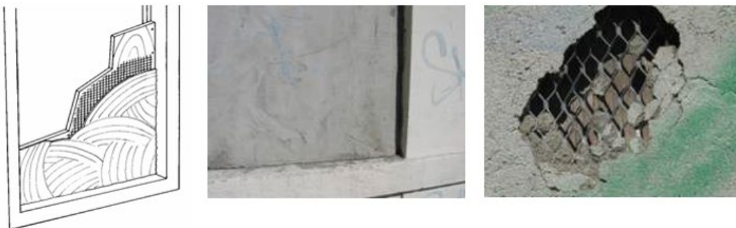
Figure 215 - Three layers forming an effective seal
