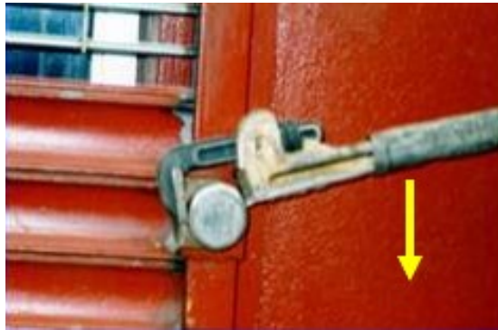
Figure 172 - Hockey puck lock with pipe wrench and cheater bar
