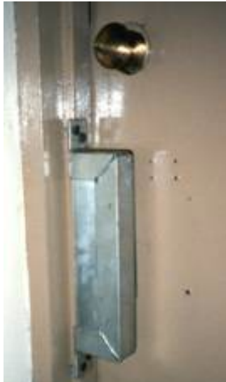
Figure 33 - Magnetic door lock add-on
