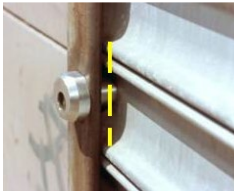
Figure 188 - Cut the body of the bolt lock
