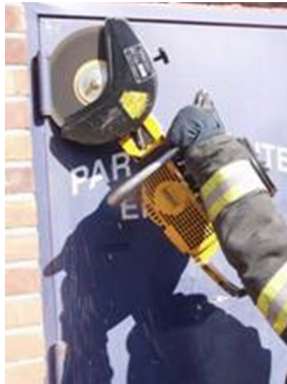
Figure 105 - Cut hinge
