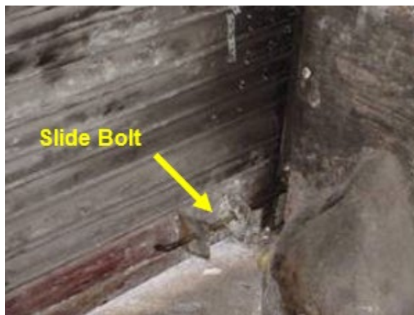
Figure 179 - Be aware of external latches that may be easier than forcing the door
