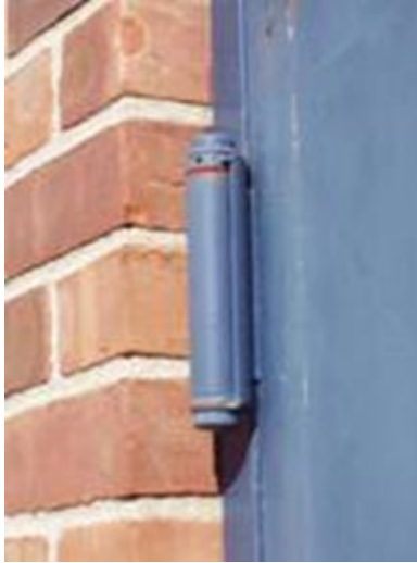
Figure 97 - Self closing hinge
