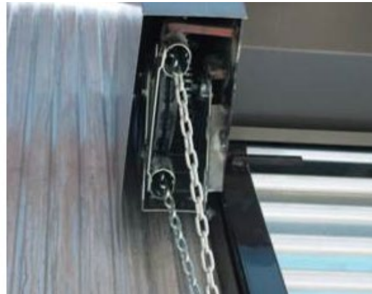
Figure 180 - Mechanical roll down gate (Chain Hoist)
