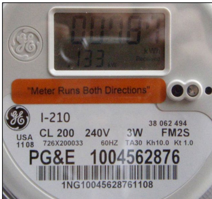
Figure 30 - Bi-directional meter labeled to indicate the presence of an alternative power source (PV).
