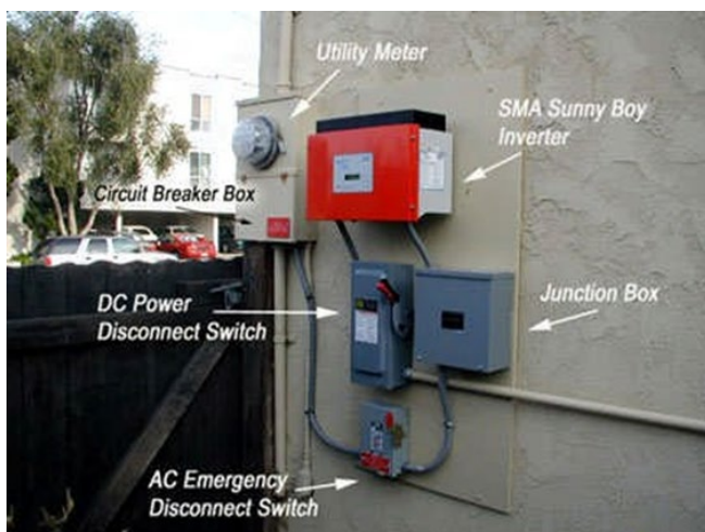
Figure 28 - Residential Solar PV inverter, DC and AC disconnect junction box and Main Electrical circuit breaker panel.
